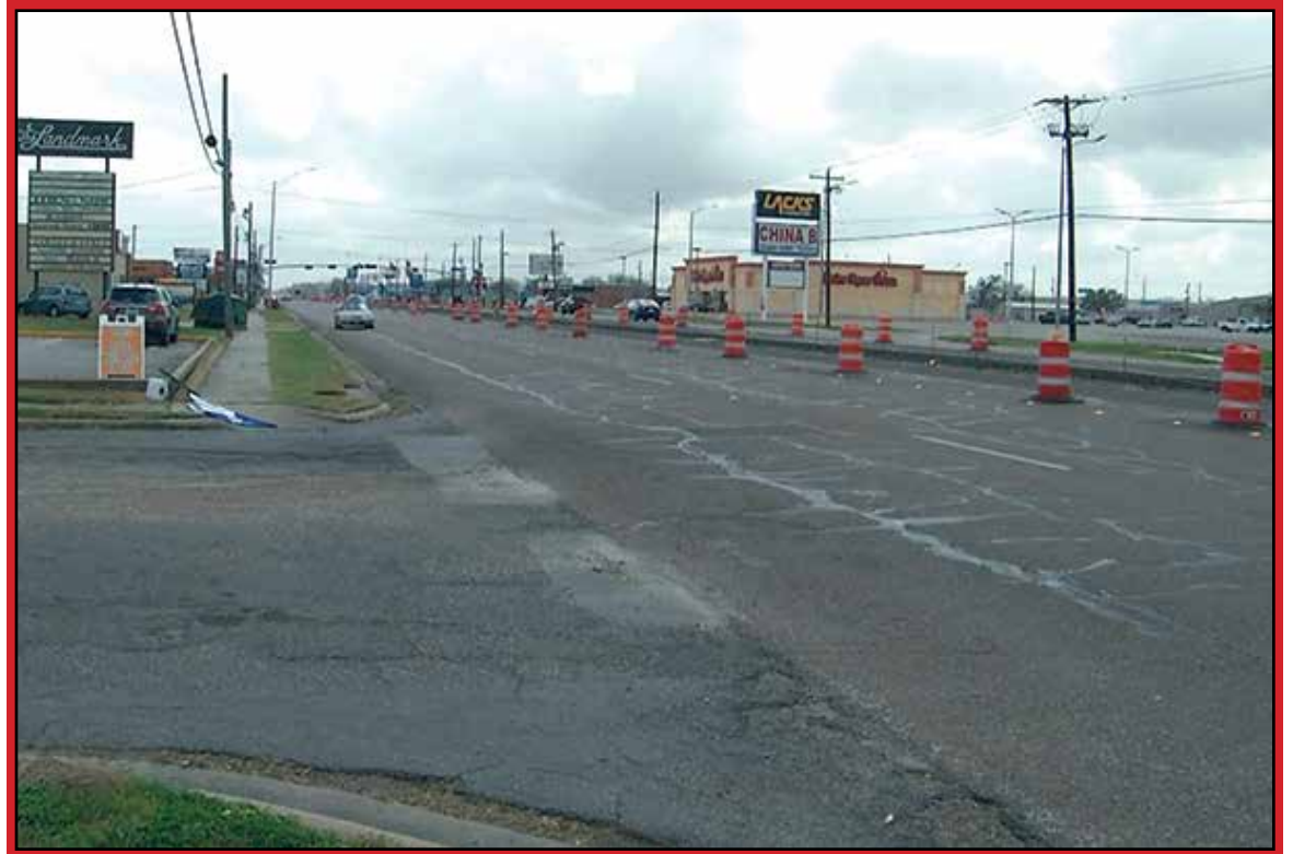
TxDOT Navarro street median project. Contributed photo.
