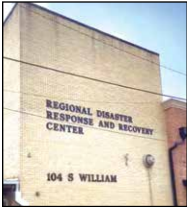
Center prepared for disaster. Contributed photo.
