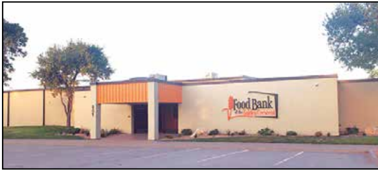
Food Bank's new location at 801 South Laurent. Contributed photo.
