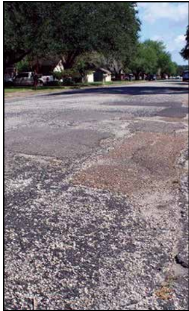
The proposed capital improvement budget for fiscal year 2023 includes utility reconstruction in part of the Tanglewood subdivision. Contributed photo.
